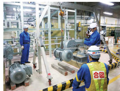
Work to dismantle and dispose of equipment related to toxic liquids (second stage work)
