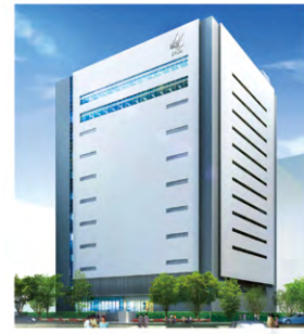
Hiroshima Data Center
