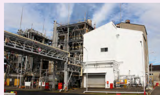
New dissolution and separation recycling facility
