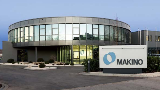
Makino Europe GmbH Headquarters (Kirchheim, Germany)
