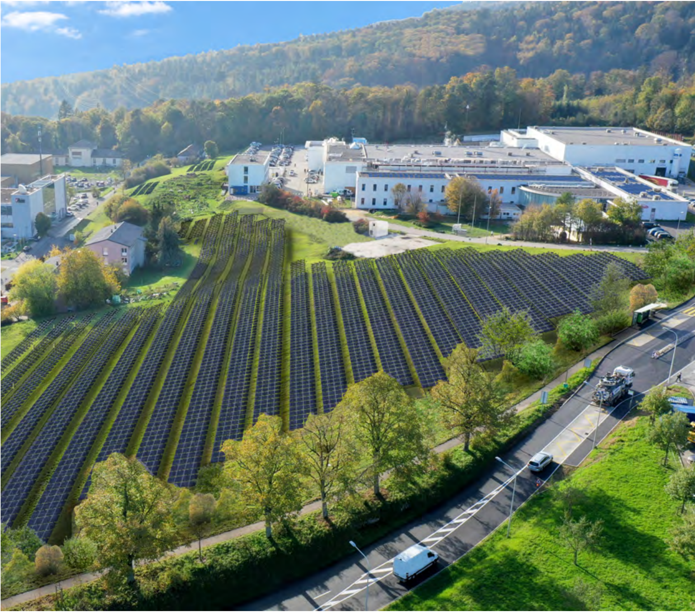
Takeda biotechnology manufacturing site in Neuchatel, Switzerland
