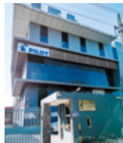
Office and factory building
