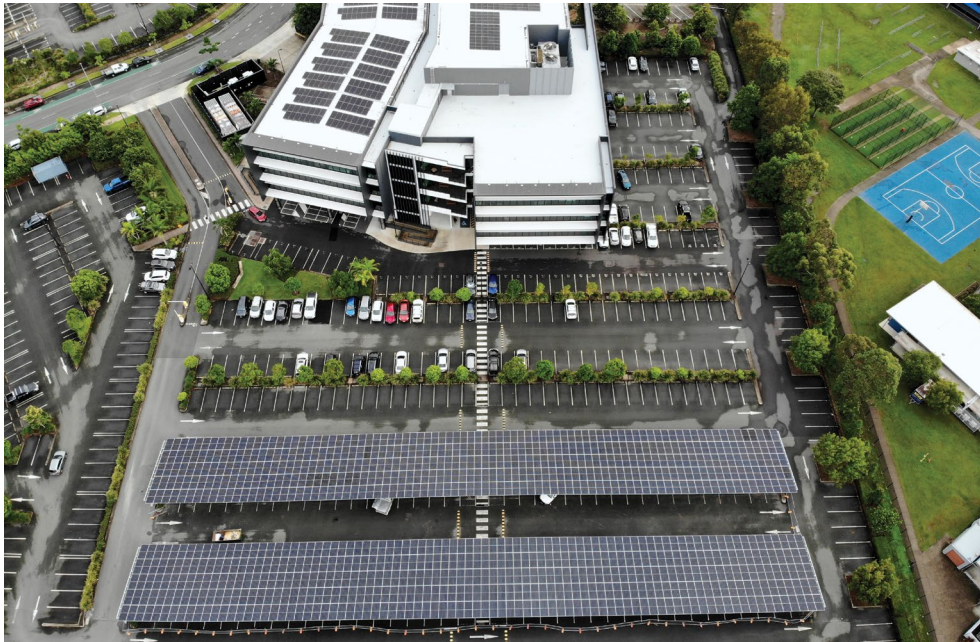
Youi solar expansion project
