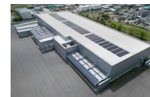
Additional solar panels installed at the Miyagi Distribution Center
