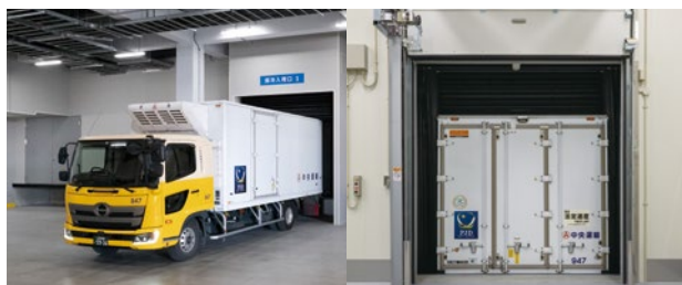
Dock shelters that prevent the intrusion of outside air through the gaps between facility openings and vehicles
