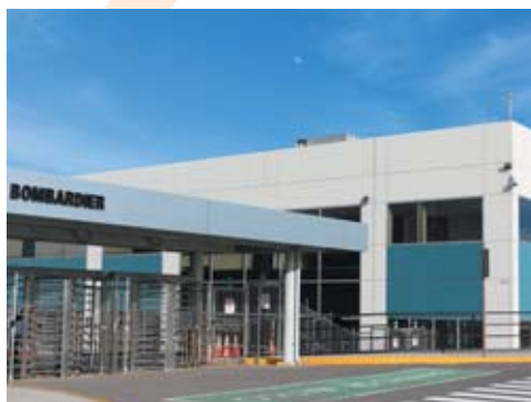
The Querétaro site specializes in the electrical harnesses and sub assemblies required for the production of EWIS systems.
