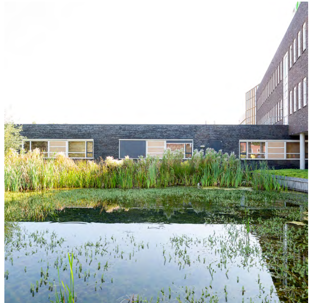
► Medical office building – Dokkum (NL)
