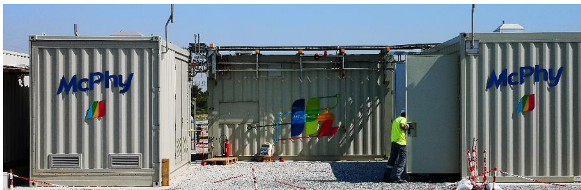
Jupiter 1000: 1 MW of electrolysis for a PtoG demonstrator in Fos sur Mer (0.5 MW alkaline + 0.5 MW PEM)
