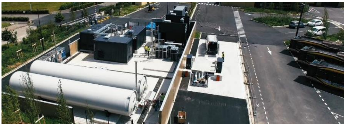
Haut de France: first zero-carbon hydrogen station for buses in France (200 kg of hydrogen / day, 0.5 MW electrolysis).
